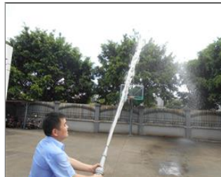
Photo of fire safety equipment Working fire hydrant.JPG
